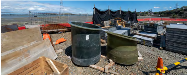
Sections of the GRP liner on site
